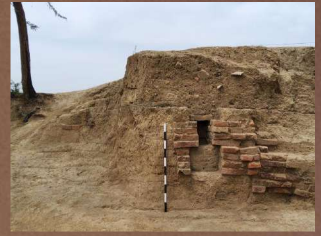
Covered Drainage System
