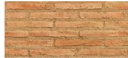
Brickwork in Lime Mortar
