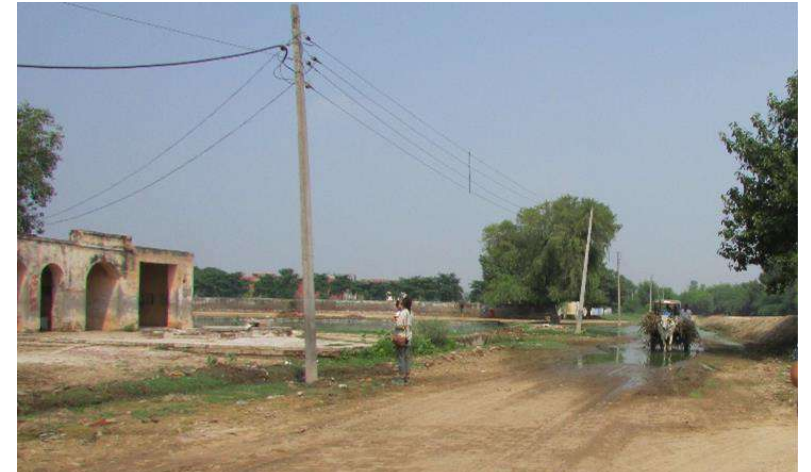
Condition of the main approach road leading to the museum near the pond
