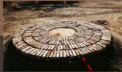
Radial Paving Base for Seating pods
