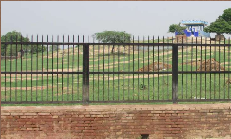
The existing Boundary wall
