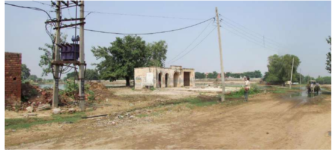
Figure 8: Existing main access road
